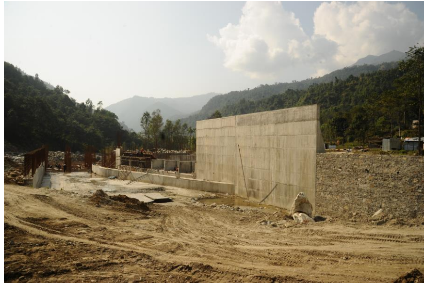
Construction of Intake and undersluice
