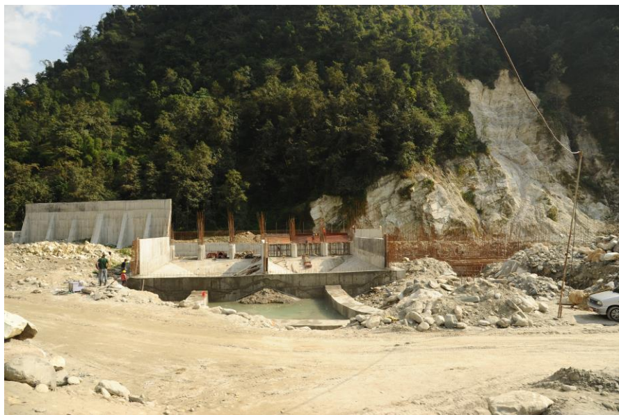
Construction of Gravel Trap
