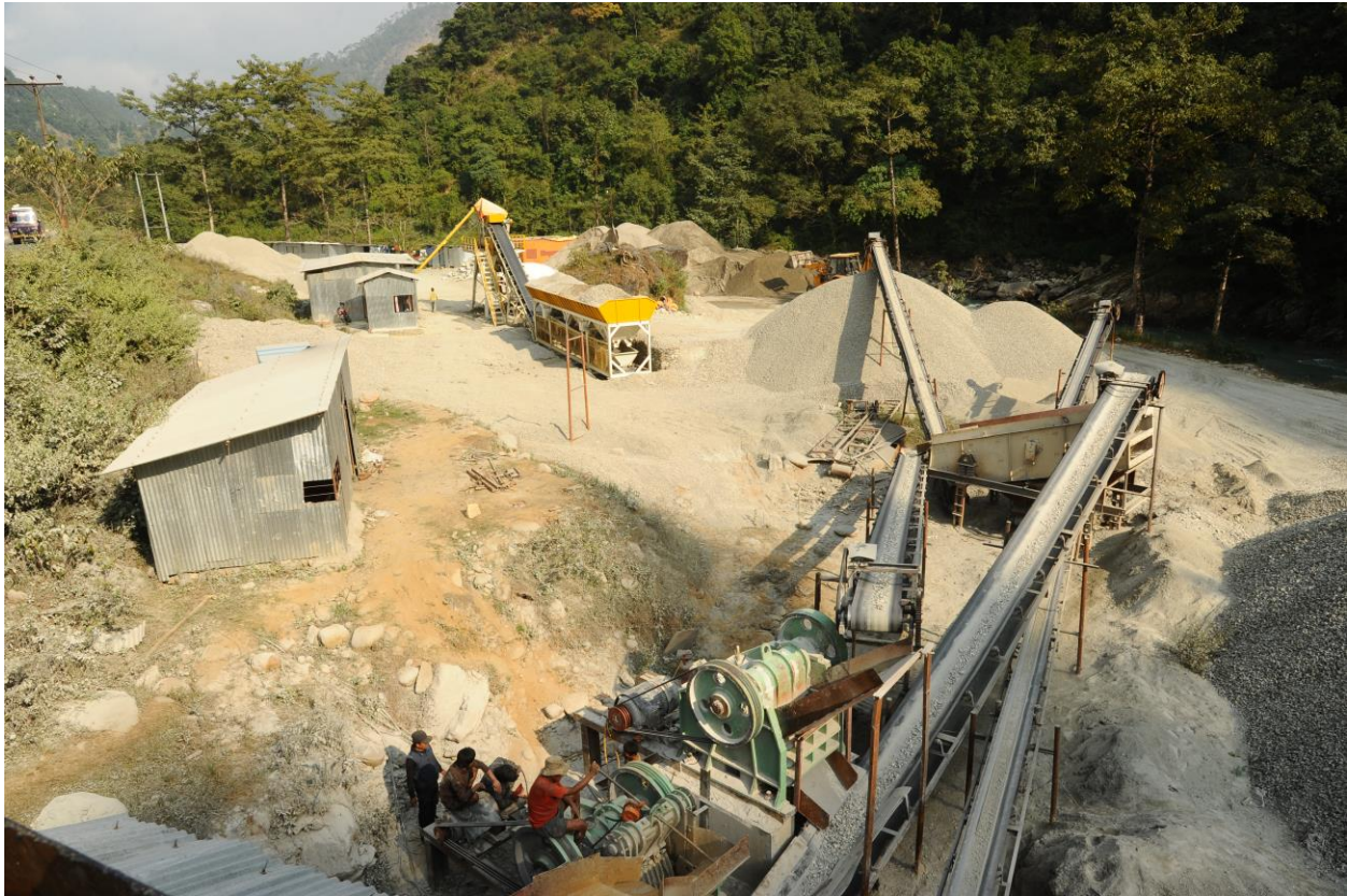
Crushing and batching plant in operation
