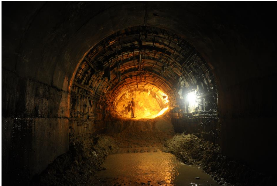
Inner view of HRT tunnel, upstream of Adit-2
