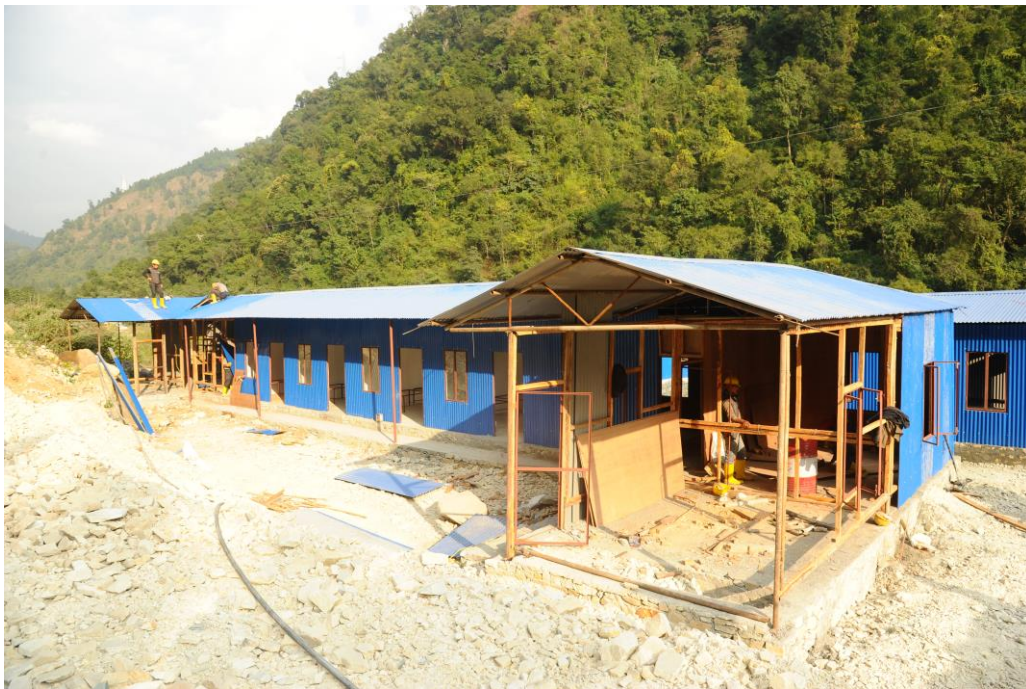
Staff quarter of South Asian Infrastructure Pvt Ltd
