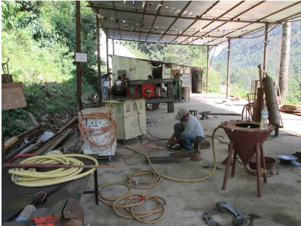
Workshop at Adit-2
