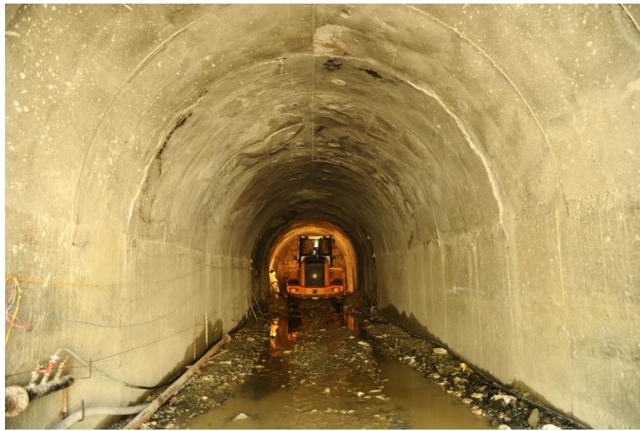
Inner view of HRT tunnel from inlet portal
