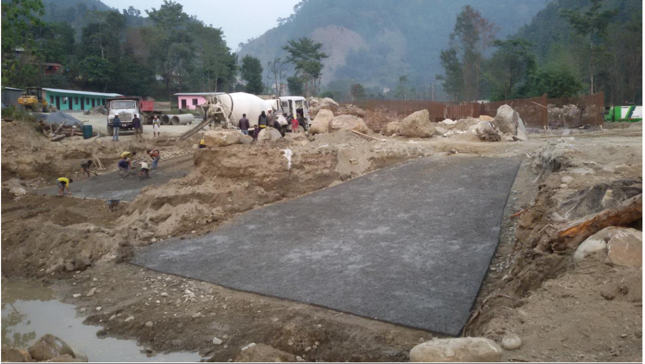
PCC at settling Basin
