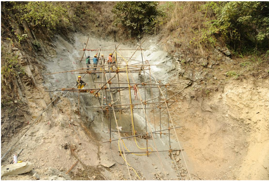
Preparation of outlet Portal
