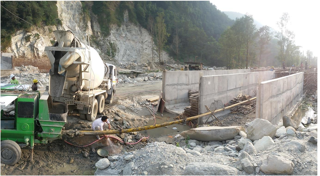
Concreting at approach canal
